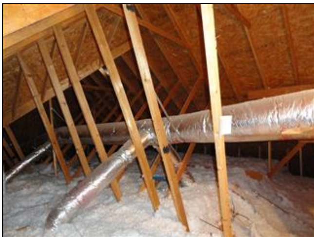
5.5 Picture 1 Attic view
