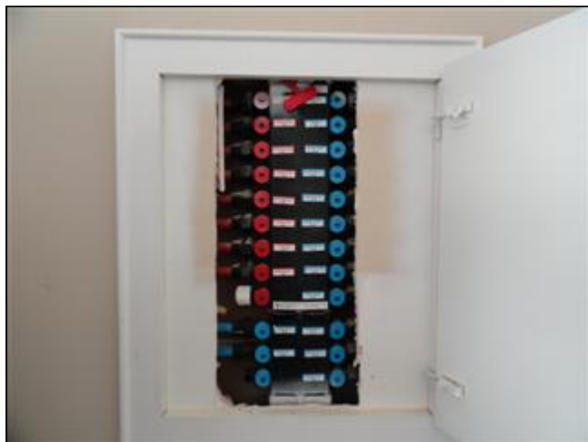
6.3 Picture 2 Water manifold in garage
